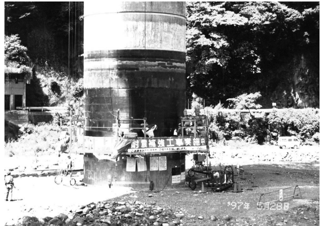
Fig. 19. Application of CFS jacketing.
