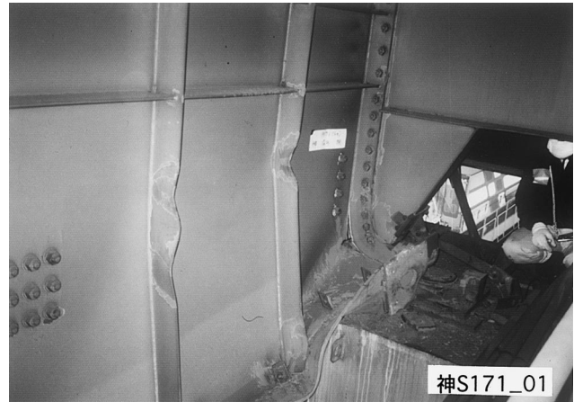
Fig 6. Buckling of main girder.
