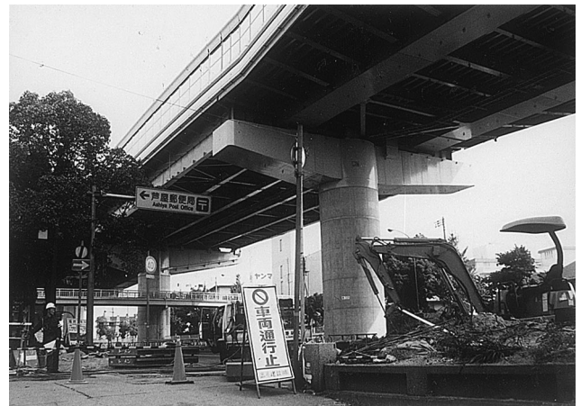
Fig. 13. After reconstruction (hybrid pier).
