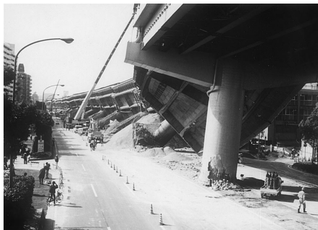
Fig. 1. Toppled columns at Fukae Section.
