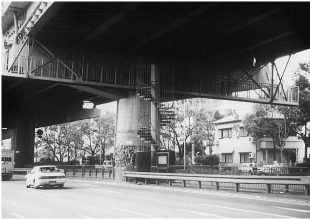
Fig 3. Damaged RC pier (ranked A).
