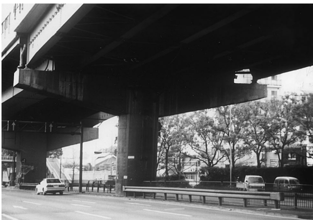
Fig 4. Damaged RC pier (ranked B).
