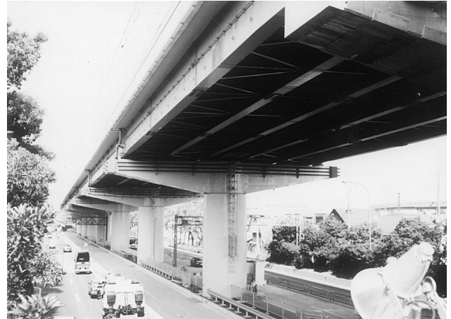
Fig 22. Strengthening of beams with external PC cables.
