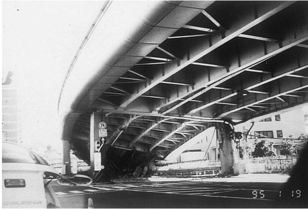
Fig. 2. Damage at Bentaen section.
