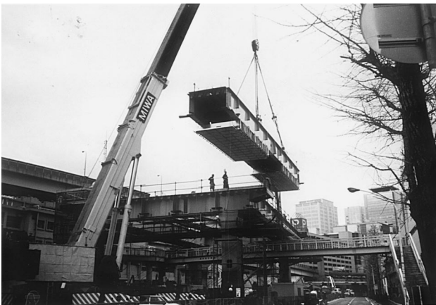
Fig. 9. Erection of main girder.
