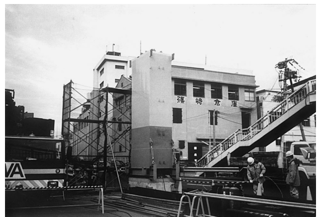
Fig. 11. Temporary stabilizer system for column.
