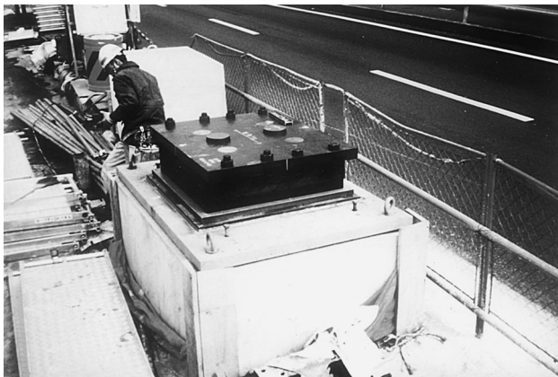
Fig. 7. Seismic isolation bearing.
