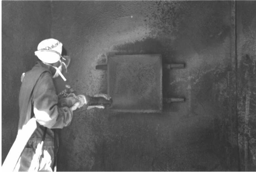
Fig. 3. Shotcreting in progress.
