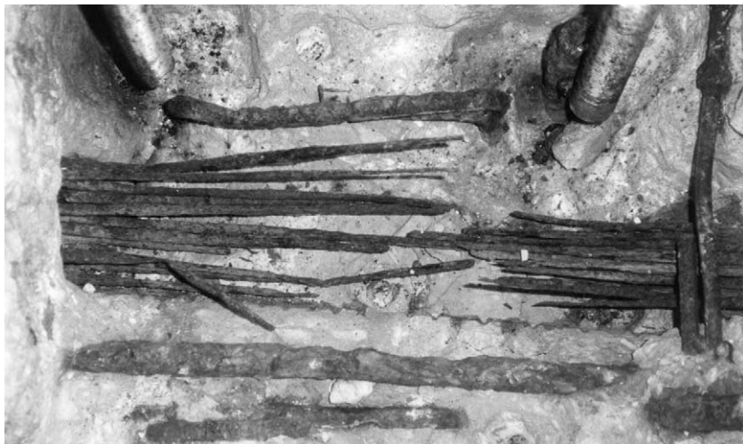
Fig. 13. Corrosion of prestressing steel in un-grouted ducts.
