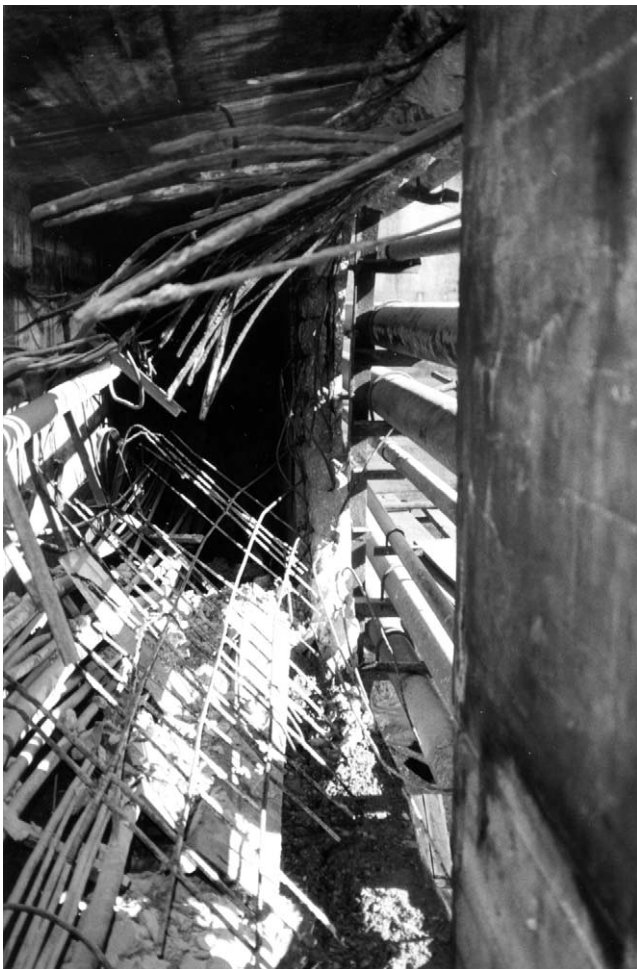
Fig. 7. Failure of the gallery wall in dock 21.
