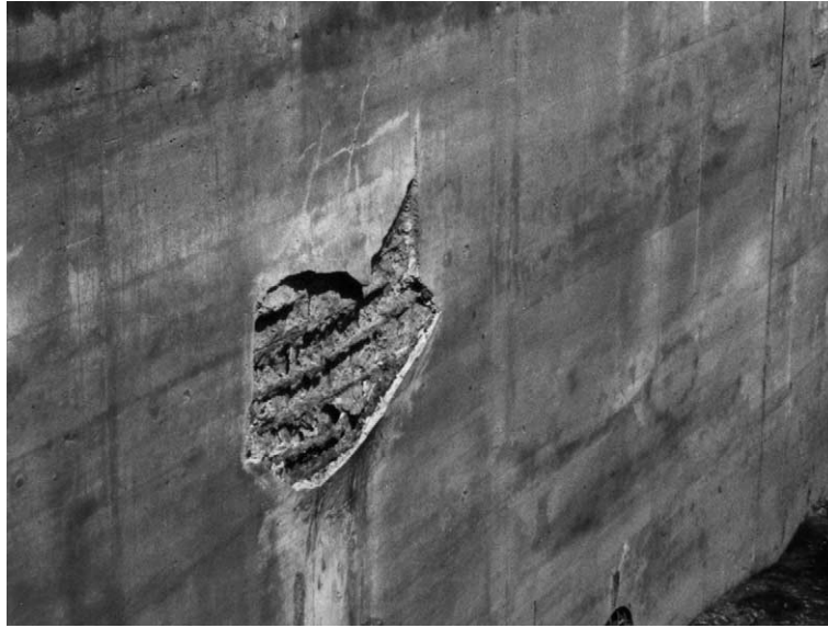
Fig. 6. Macro corrosion cell in dock 22 walls.
