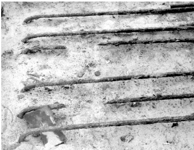
Fig. 11. Bars with 25 mm diameter totally corroded.
