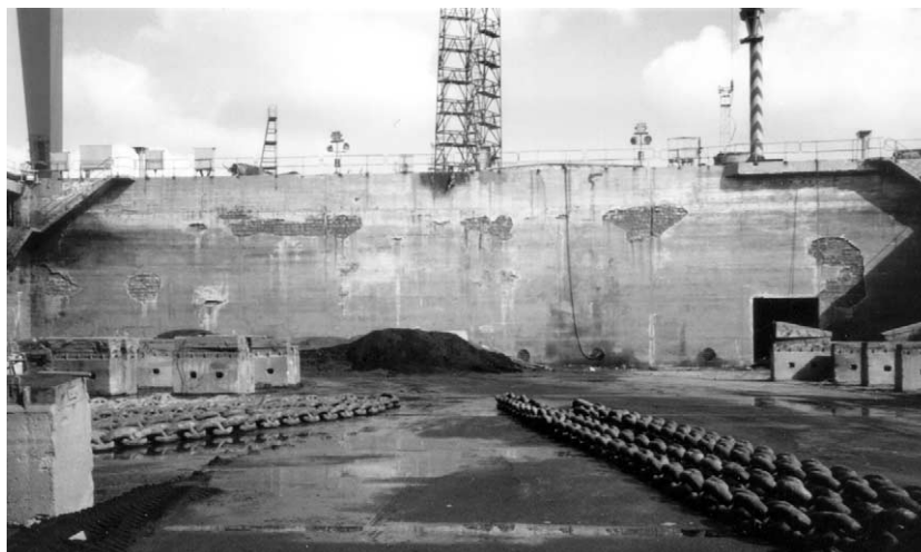
Fig. 5. Deterioration of the northern wall of dock 22 (1999).
