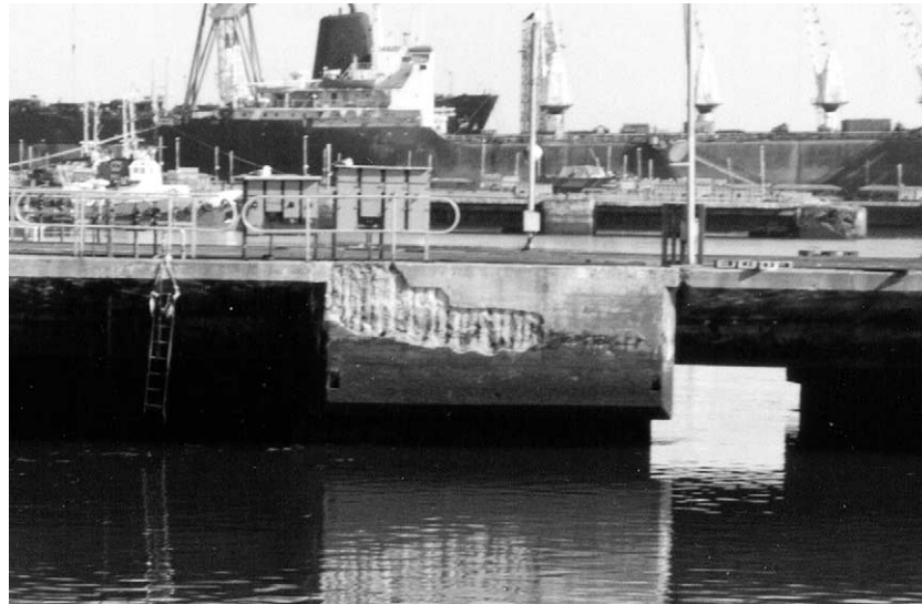
Fig. 10. Typical deterioration observed in the splash and tidal zones.
