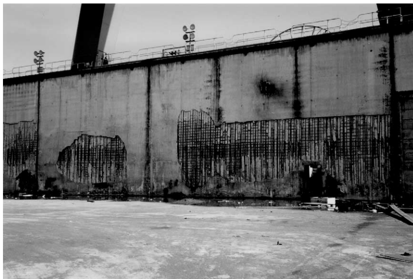
Fig. 3. Typical deterioration of dock 20 walls after 10 years of exposure.
