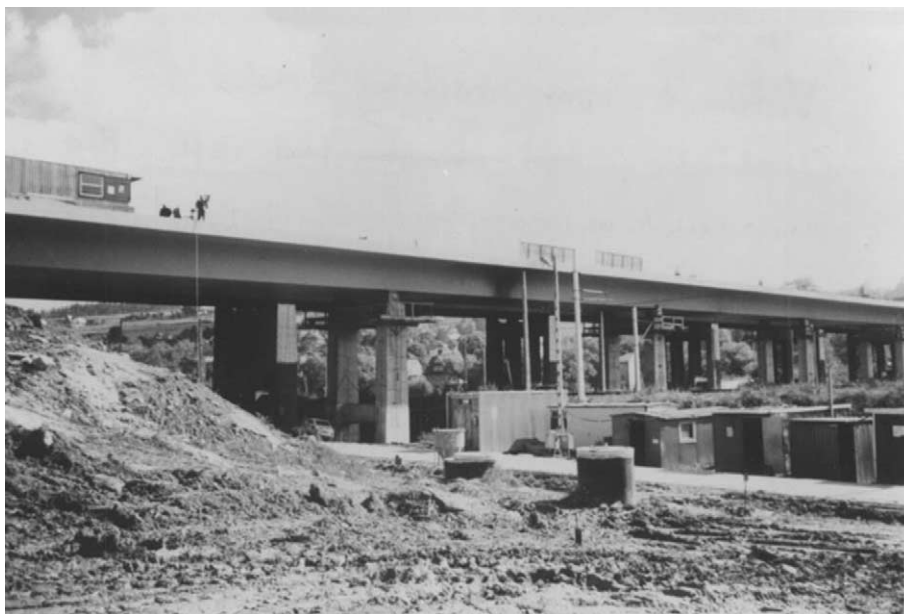
Fig. 2. Viaduct over railway trucks in Chabowka with superstructure from concrete class B60.
