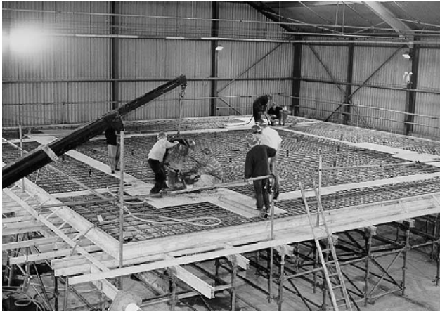
Fig. 1. Reinforcement placement and casting of columns prior to slab concreting (courtesy of Taywood Engineering Ltd.).
