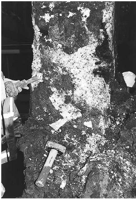
Fig. 1. Severe TSA at the base of a 29-year-old bridge column exposed to wet, reworked Lower Lias Clay.
