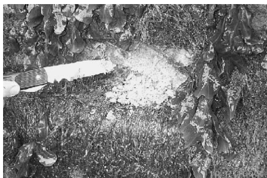
Fig. 6. Degraded friable mortar sample on site equivalent to sample 13 described here.
