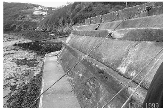
Fig. 5. Mass concrete from harbour structure from which sample 11 was collected within the inter-tidal zone.
