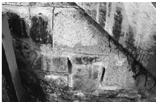
Fig. 1. General view of harbour wall steps. The SRPC bedding mortar is being severely eroded from the area under the limestone facing.
