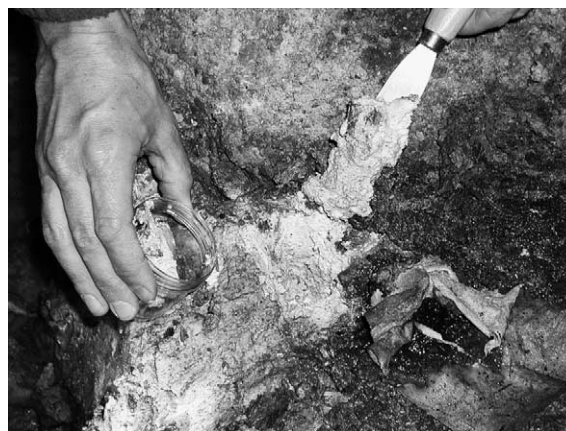
Fig. 6. Portion of the base of the tunnel lining with the drain channel to the left. Large volumes of concrete have been altered into a soft mush like or crumbly material depending on the degree of water saturation. The concrete deterioration is limited locally to volumes of several dm 3 and was triggered by permeable pathways through the concrete. Some years after construction of the tunnel the drainage system collapsed, the pressure of the ground water increased and percolating water was forced to penetrate the unprotected concrete lining of the tunnel.
