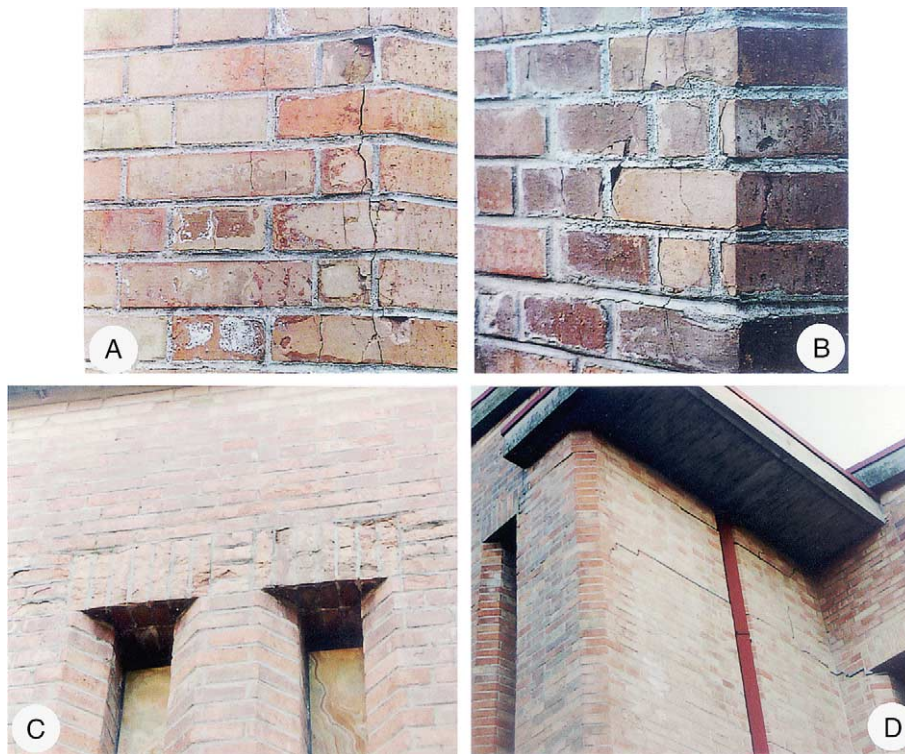
Fig. 2. Decay aspects of the brickwalls (see text).
