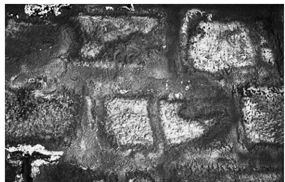
Fig. 1. Inappropriate consistency and application of repair mortar covering. It can be seen that the layer of repair mortar covers not only the joints but also the limestone blocks. Development of the reaction is best seen in the lower left corner of the figure.
