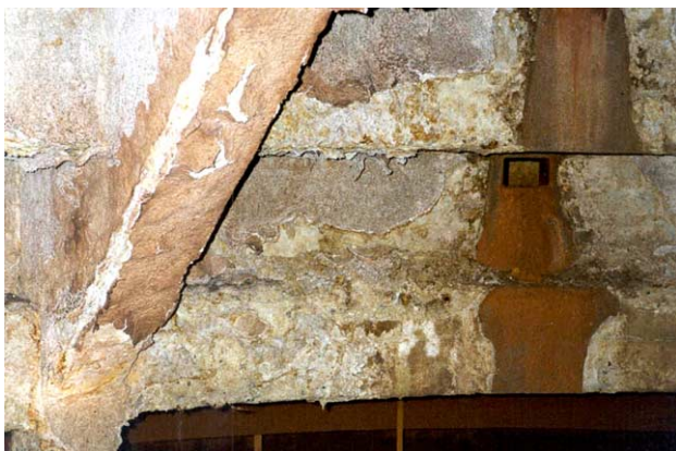
Fig. 1. Concrete ‘dome’ with surface spalling, below the oxidation stairs.
