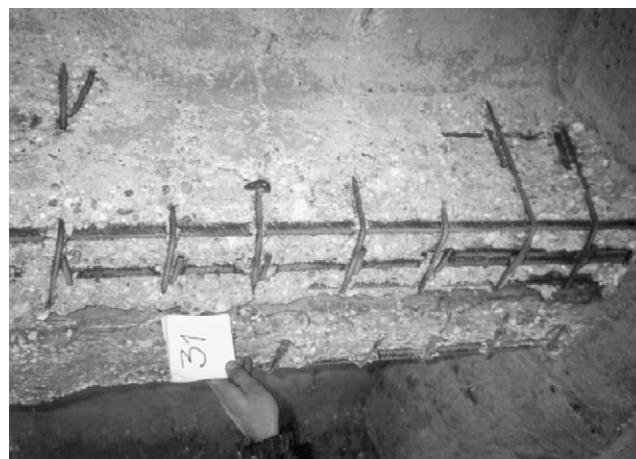
Fig. 4. A typical damage of the concrete—3.
