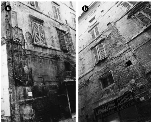
Fig. 1. Deterioration of the rendering mortar caused by ettringite (a) and thaumasite (b) formation in a building located in the historical centre of Ancona.
