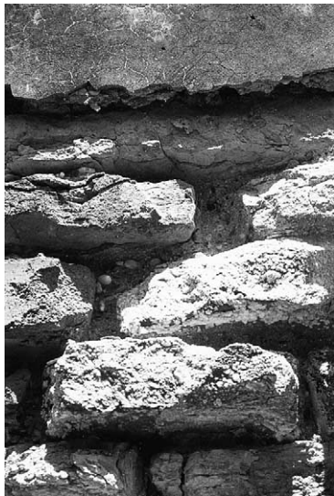
Fig. 5. Deterioration of rendering mortar of the Vanvitelli's Mole.
