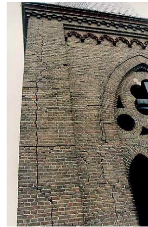
Fig. 6. Church tower (Noordwijk), case study 2, with both vertical and horizontal cracks.
