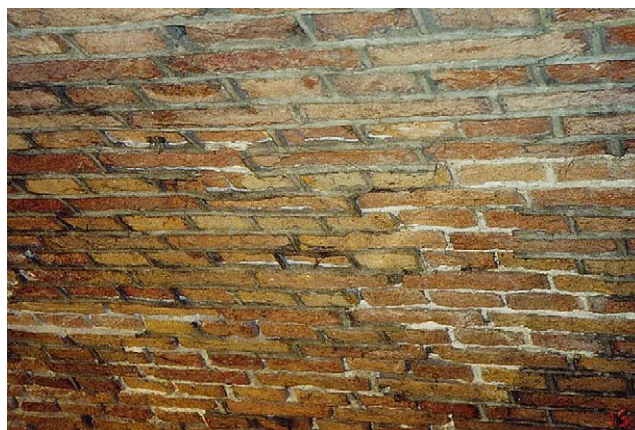
Fig. 2. Damage to masonry in vault intrados (case study 1).
