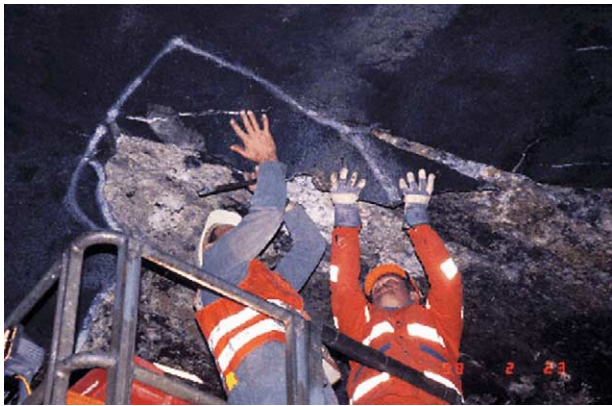
Fig. 1. Location 42/154 with larger areas of loose shotcrete (dark due to a soot layer on the surface) and parts of the lining already broken off. Dripping ground water could be sampled on the clean masonry behind the technicians.
