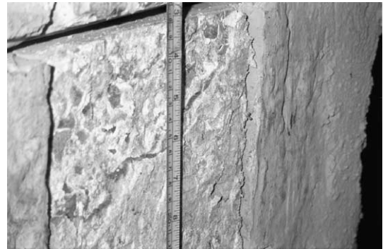
Fig. 1. Breakout of concrete to column with TSA showing white pasty surface at 5 mm depth and white 'halos' around aggregate at 10 mm depth.
