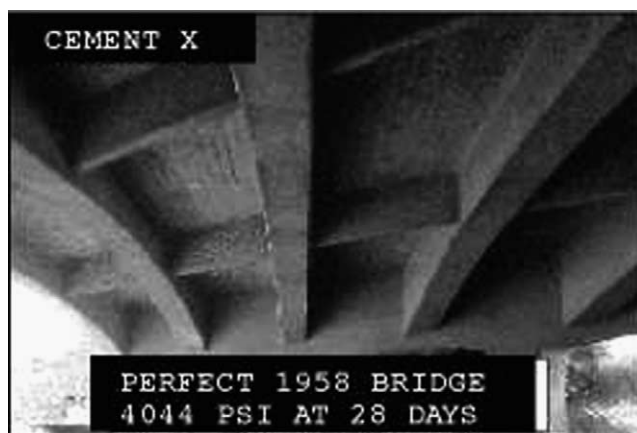
Fig. 3. Cement X was a slow-hardening Portland cement typical of the low-crack North American cements of 1954. Some form marks, not cracks, are visible.
