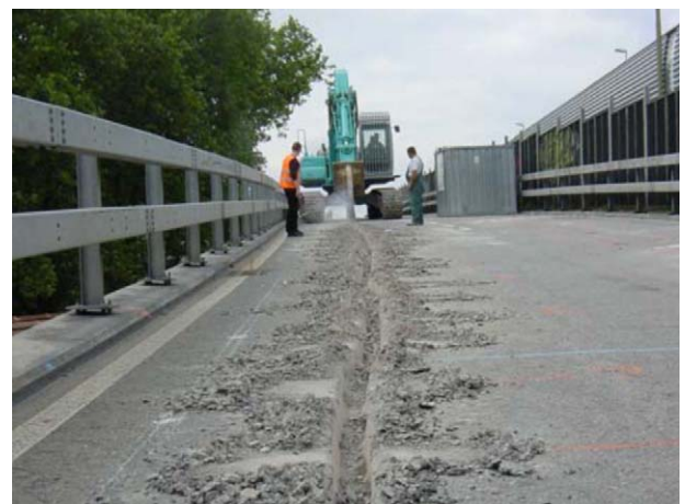
Fig. 22. Pavement opening with excavator.
