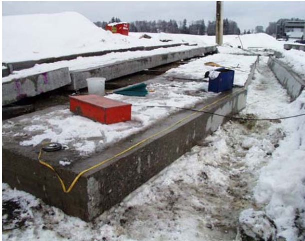
Fig. 19. Sawed bridge deck.
