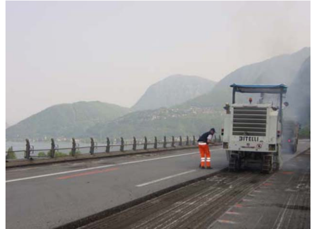
Fig. 21. Pavement removal with milling machine.
