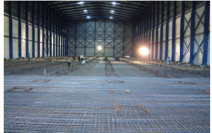
Fig. 2. Overall view of slab reinforcement ( \varnothing 16 \text{ mm}/0.15 \text{ m} ).
