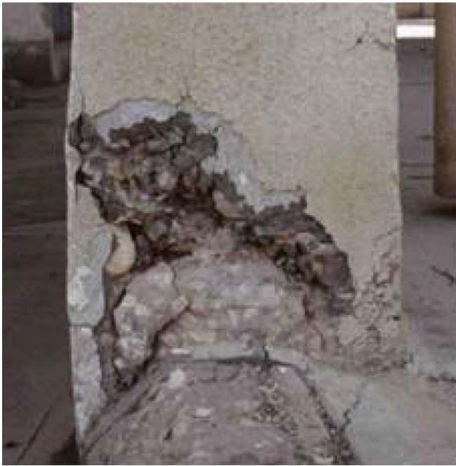
Fig. 1. Deterioration of columns in the Arabian Gulf region.
