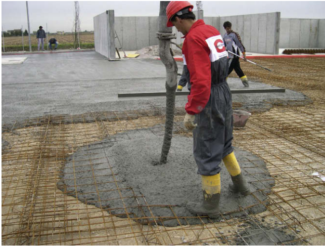
Fig. 7. Placing of the concrete mixture at a superfluid consistency (slump = 230 mm) for a reinforced industrial floor.
