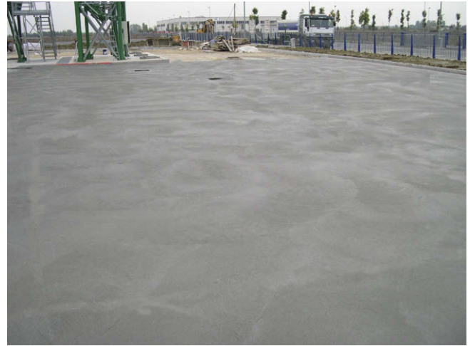
Fig. 10. View of the concrete floor area without contraction joints.
