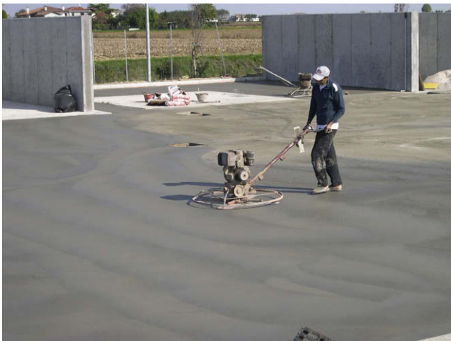
Fig. 8. Finishing operation of the concrete floor.
