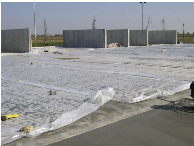
Fig. 9. Protection of the concrete floor after finishing for 1 day from placing.
