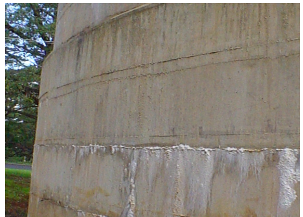
Fig. 6. General view of the Bowral water tank with efflorescence from a joint.
