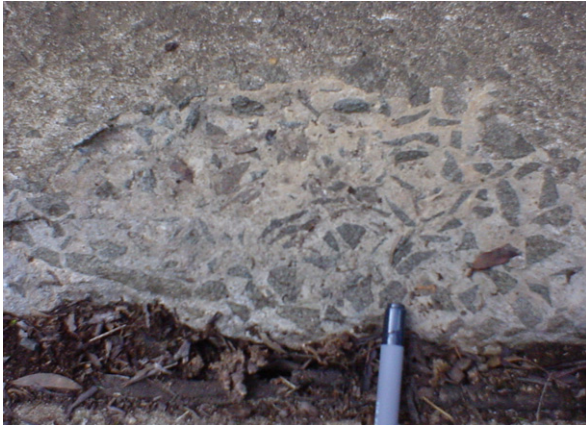
Fig. 7. Exposed aggregate at base of water tank.
