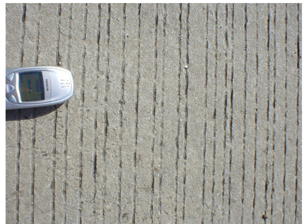
Fig. 11. Road shoulder built with Nattai River Cut 5 aggregate, free of cracks and staining.
