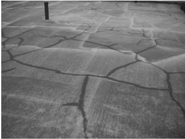
Fig. 1. Early age cracks, occurrence within the first 4 h after casting, crack spacing approximately 1 mm.
