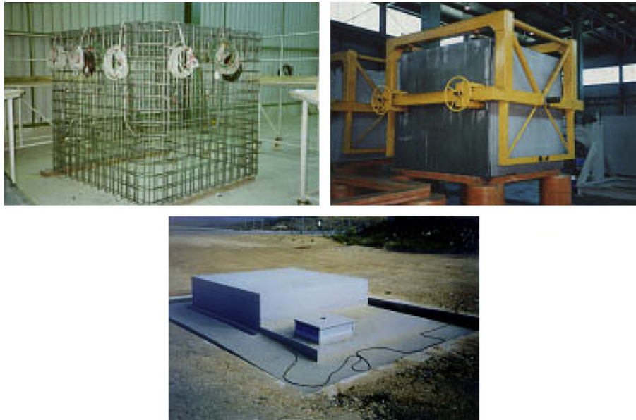
Fig. 6. Various stages during the embedment of sensors inside the pilot container in El Cabril, Córdoba.
