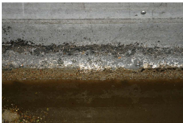
Fig. 1. Evidence of corrosion in grit removal tanks with gypsum and exposed aggregate visible above the water line in a wastewater treatment plant constructed in 2003.
