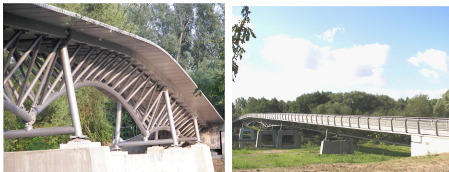
Fig. 1. Gaertnerplatzbridge in Kassel, under construction (left) and in use (right). Girders and deck plates made of UHPC are glued with an epoxy resin. Slab thickness is only 85 mm.
