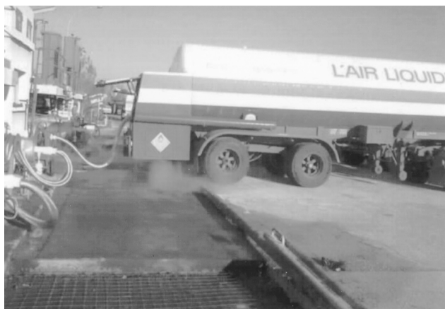
Fig. 10. Examples of applications for industrial floors: aluminum factory (advantage of CAC, resistance to thermal shock), factory producing earth-moving vehicles (advantage of CAC, resistance to abrasion), and cryogenic filling station (advantage of CAC, resistance to thermal shock).
