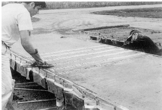
Fig. 7. A photo of the tubes embedded in the top surface of the deck [3].
