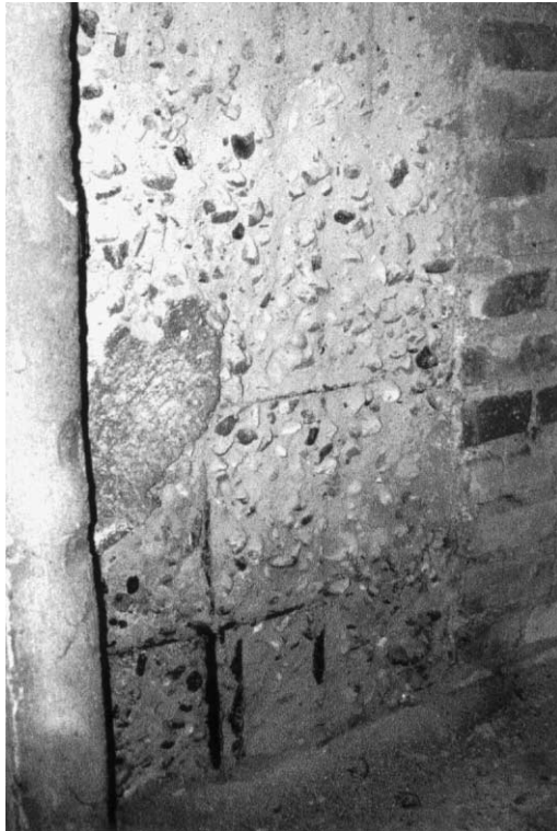
Fig. 1. Example of severe degradation of concrete and steel reinforcement of the building foundations: P 2 pier.
