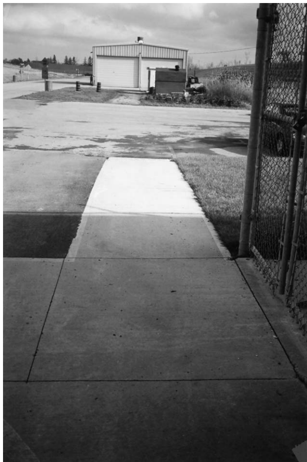
Fig. 4. Section of an experimental concrete sidewalk incorporating 50% WLP as partial replacement for mixing water.
