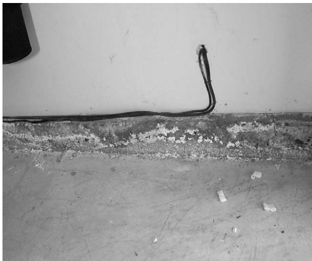
Fig. 2. Sulfate crystal formation and scaling damage on stem wall.
