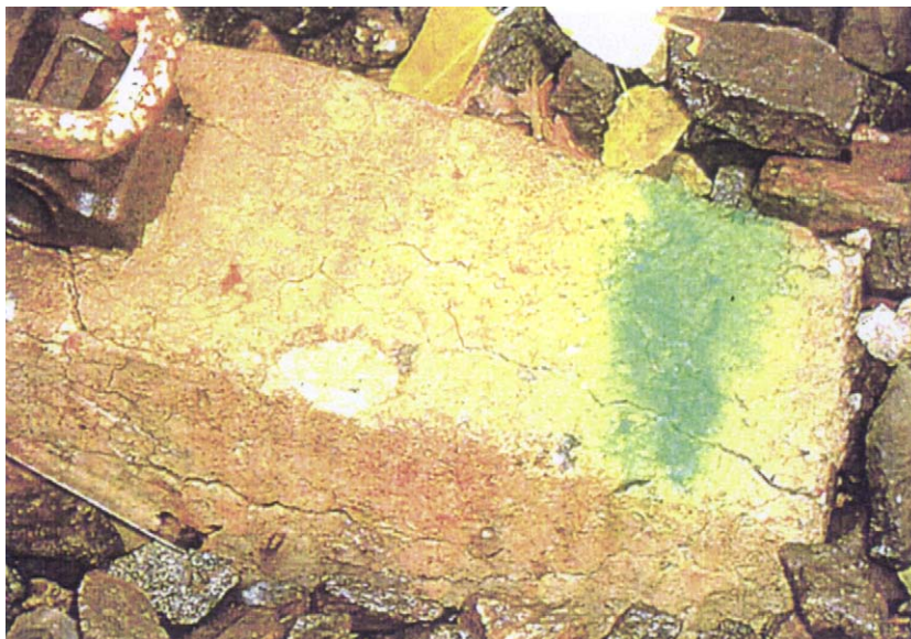
Fig. 1. Map cracking on the shoulder of a railroad tie.
