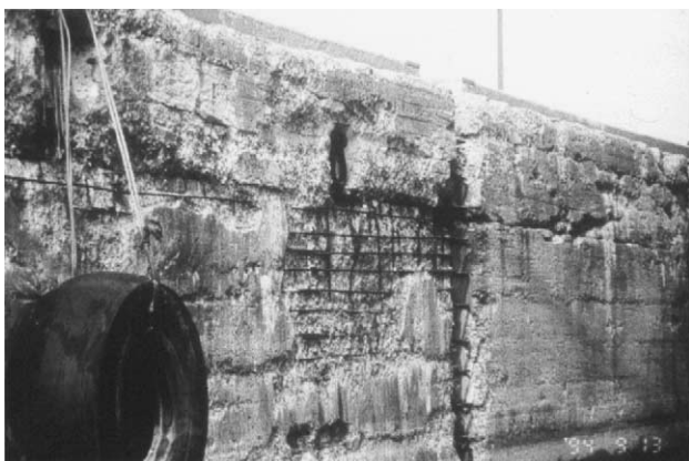
Fig. 2. Photograph of typical scaling damage of Wharf 105.
