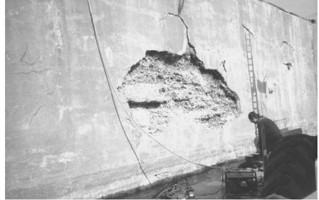
Fig. 11. Photograph of typical damage of Wharf 45 showing the bad anchoring of previous repair concrete.
