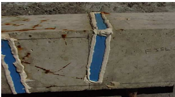
Fig. 4. Cracks protection.
