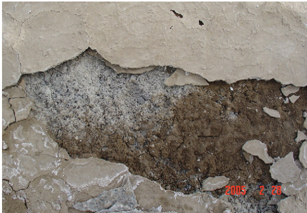
Fig. 1. The photo of the attacked concrete.
