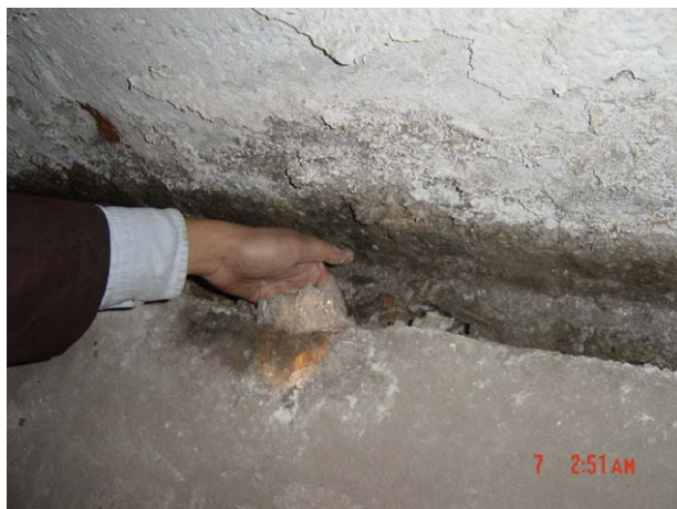
Fig. 4. Deterioration in the tunnel drainage channels.
