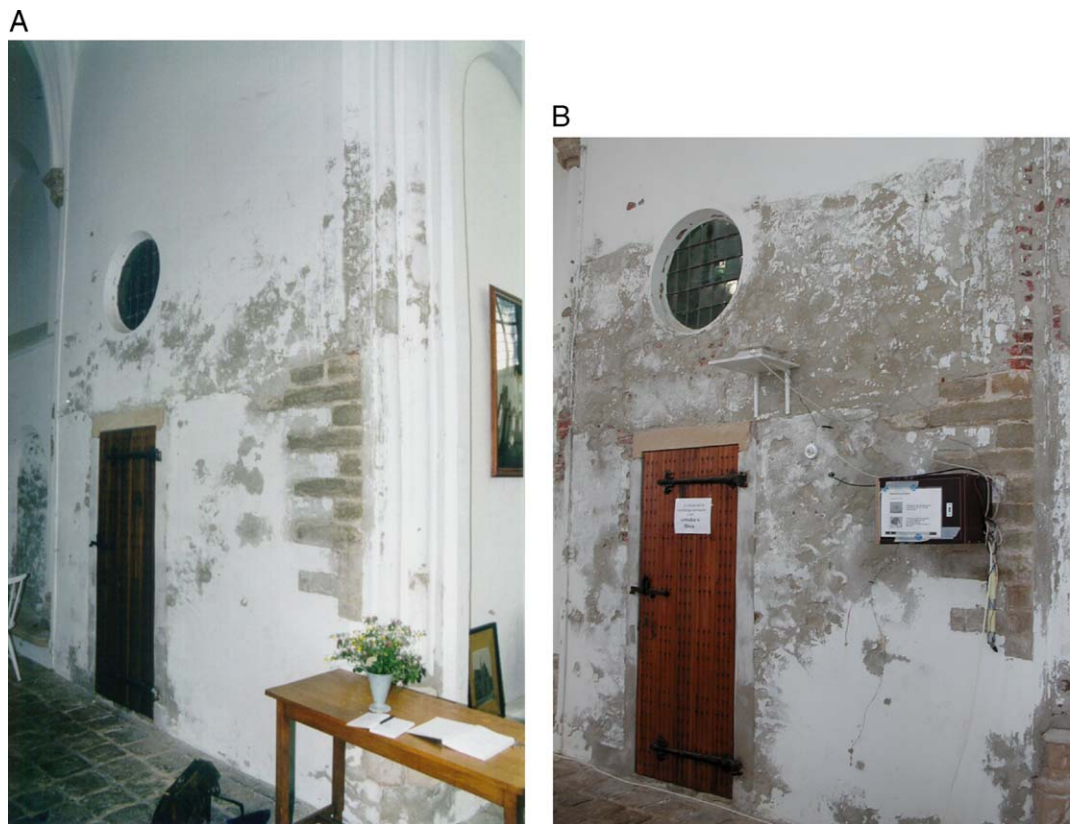
Fig. 12. Evolution of the damage in the years 2000 (left) and 2004 (right) (St. Nicholas Church, Brouwershaven, The Netherlands).
