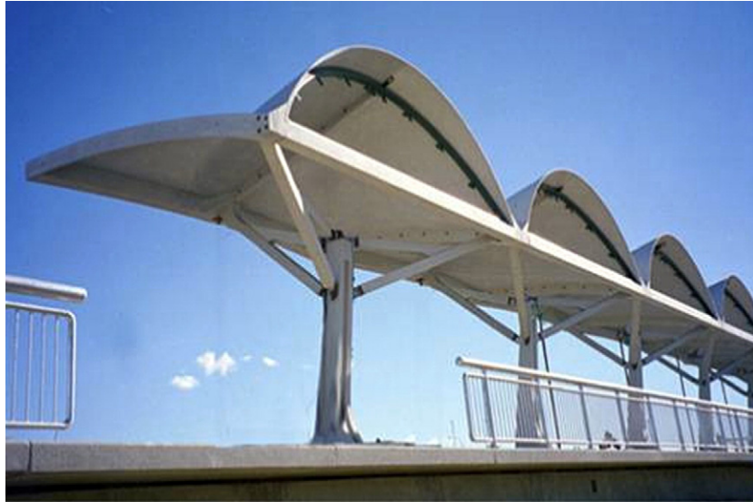
Fig. 5. LRT Train Station (Calgary, Canada): 24 thin-shelled Ductal®-FO canopies (architects: CPV Group Architects & Engineers Ltd; photo: Courtesy ARR Medialibrary Lafarge).
