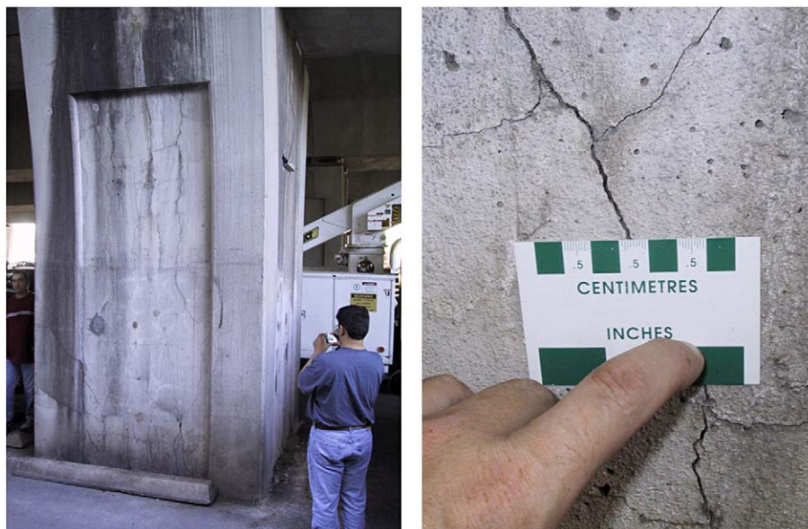
Fig. 1. Typical appearance of columns after approximately 15 years.
