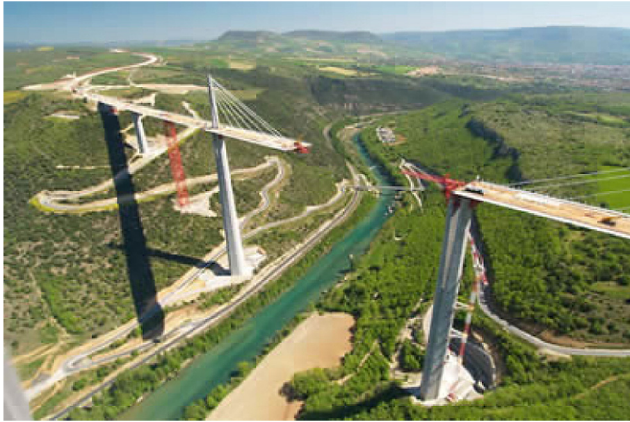
Fig. 1. The Millau viaduct, during the building of which 53,000 m 3 of the concrete used as a reference concrete in this paper were cast.
