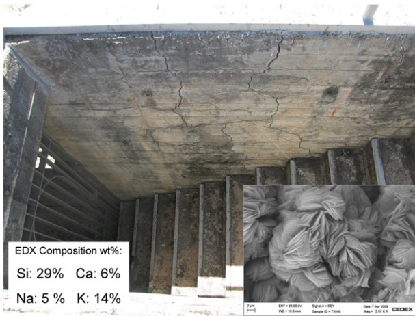
Fig. 1. Aggregate C was extracted from a dam affected by ASR. SEM–EDX confirms that expansion and cracking of concrete are due to alkali silica reaction.
