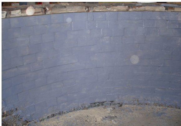
Fig. 5. Photograph of frit coated MgO–C brick of working lining in steel ladle after brick installation but before use.
