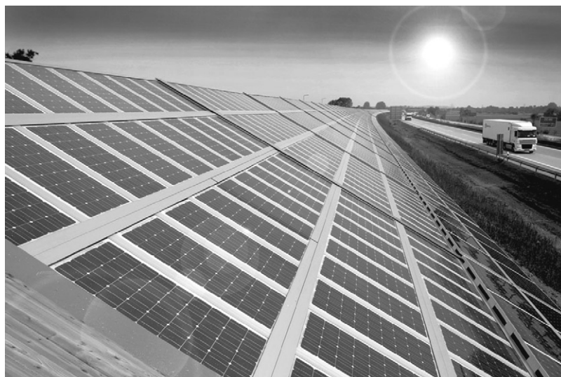
Fig. 10. Panel of porcelain tiles fitted with photovoltaic cells.
