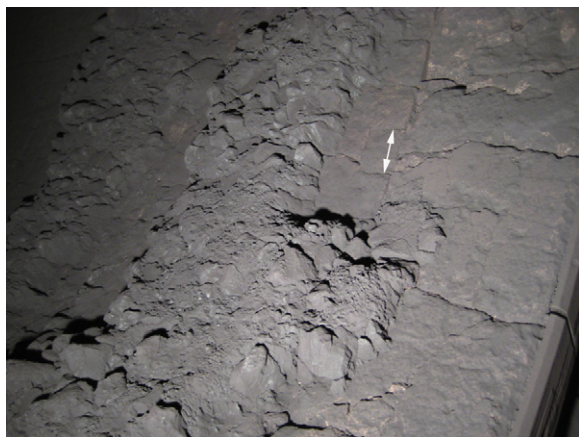
Fig. 1. Photo showing deposits in the kiln KK2, Kiruna, Sweden, June 2010. The white arrow in the image marks the brick width, which is 17.5 cm.
